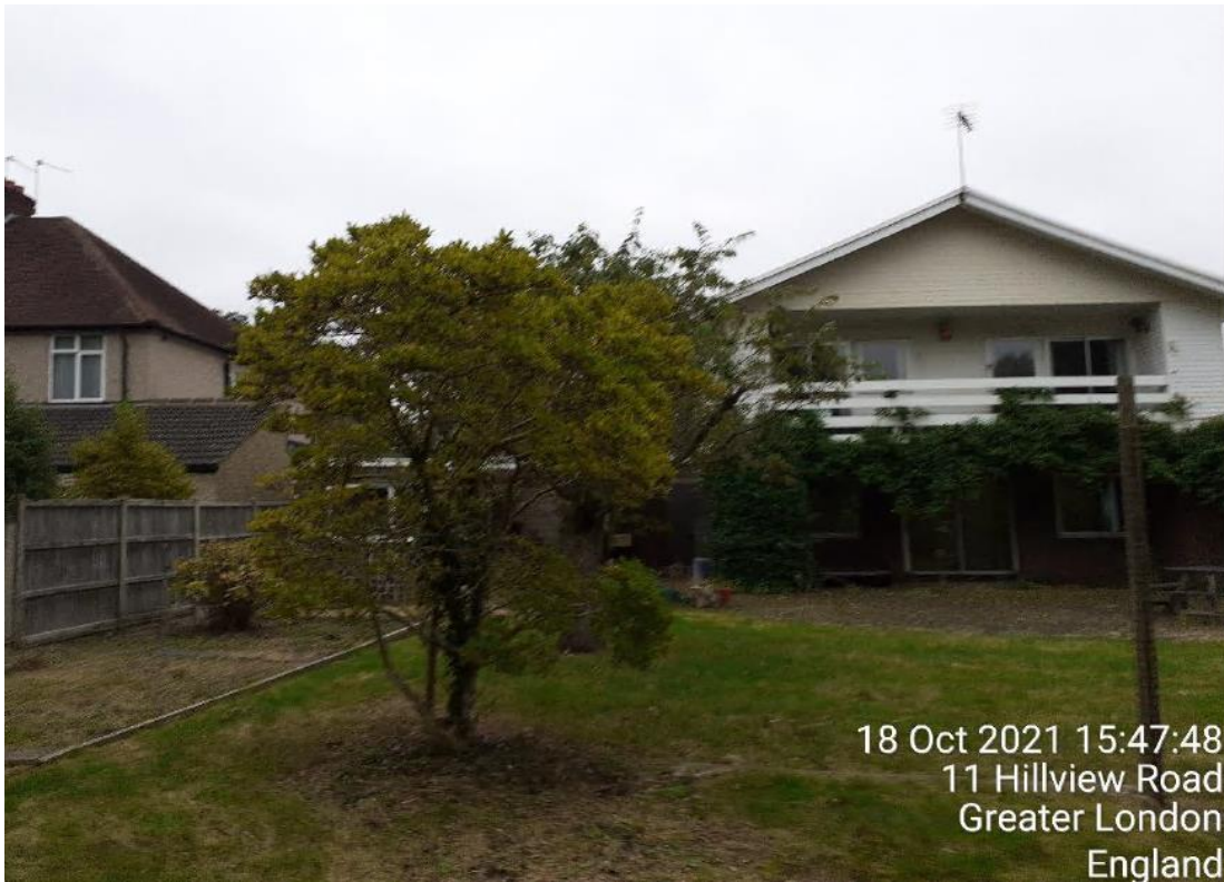
Rear boundary and garage
