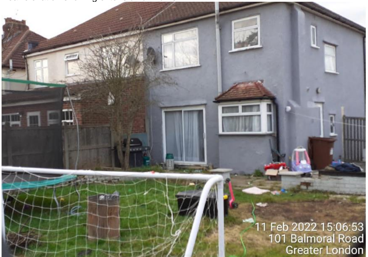
Rear elevation showing extension at No.18.
