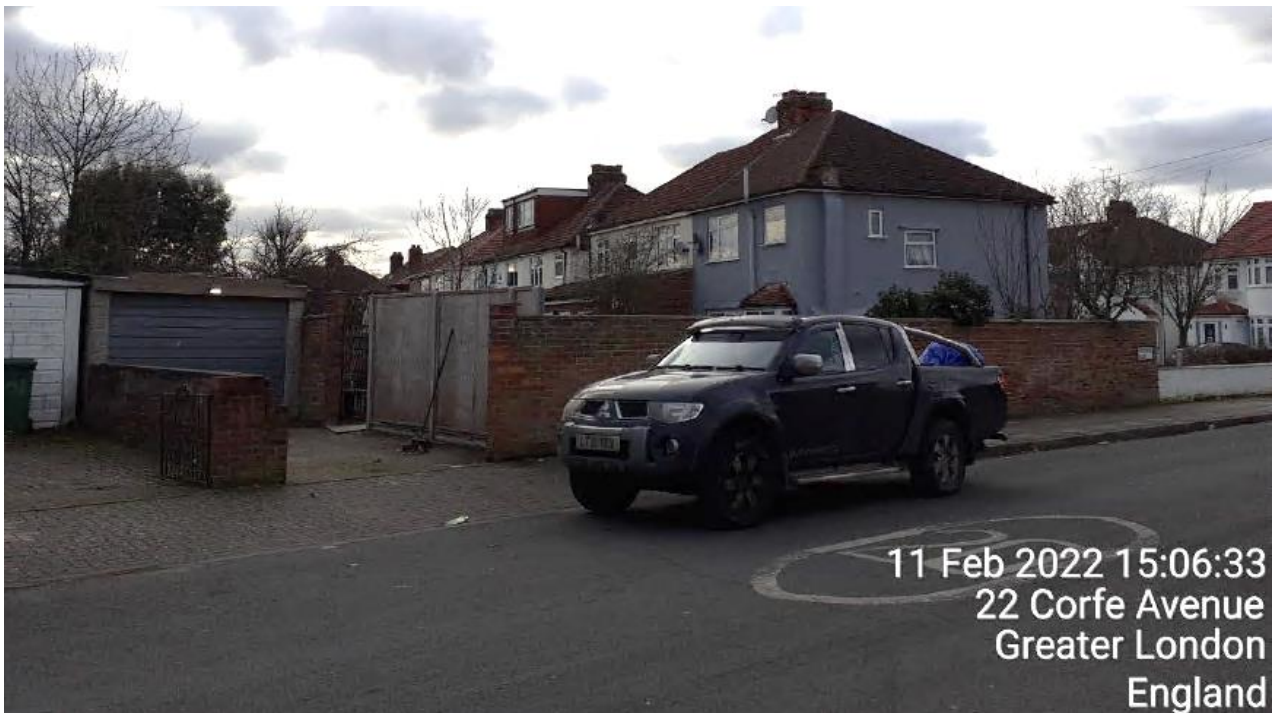
Rear boundary and garage
